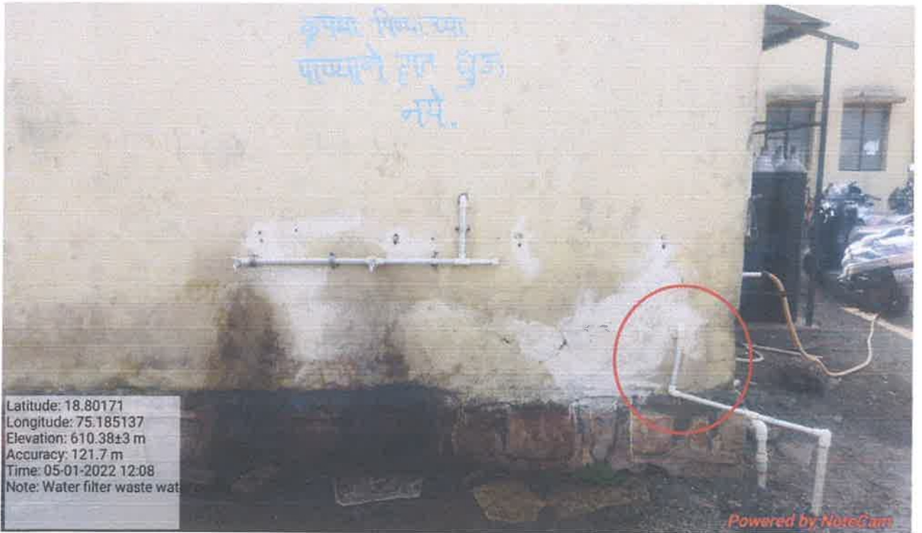
Water filter waste water outlet
