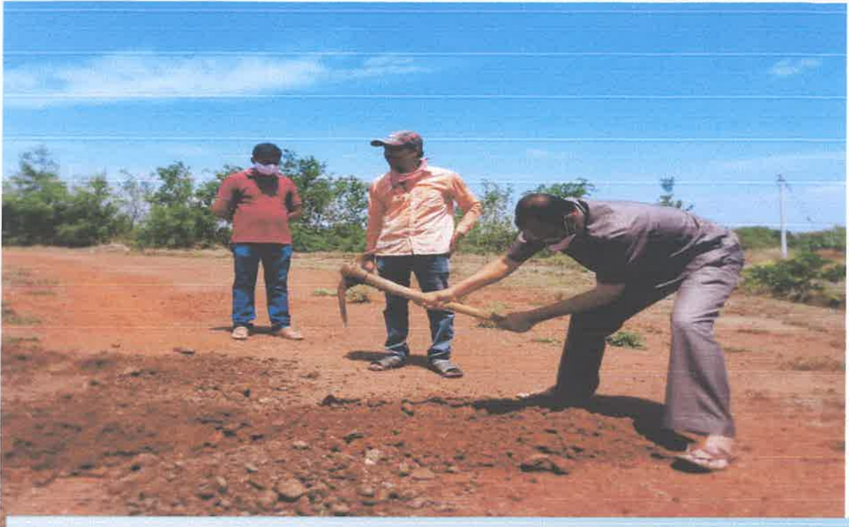
Disposal Pit for Bio-medical Waste
